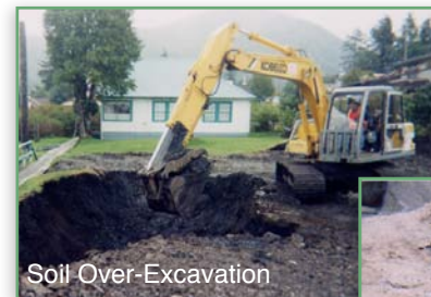
Remedial System Construction
