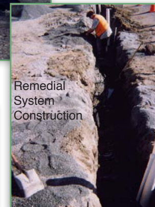
Soil Over-Excavation
